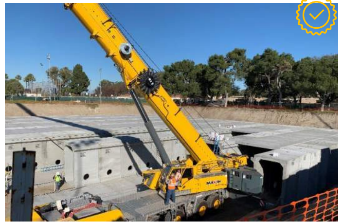
Craftwater Engineers led the development of the most innovative stormwater capture facilities in the GWMA. Mayfair Park SW Capture Project incorporated pretreatment, filtration discharge, and sanitary sewer discharge for optimal system performance.
