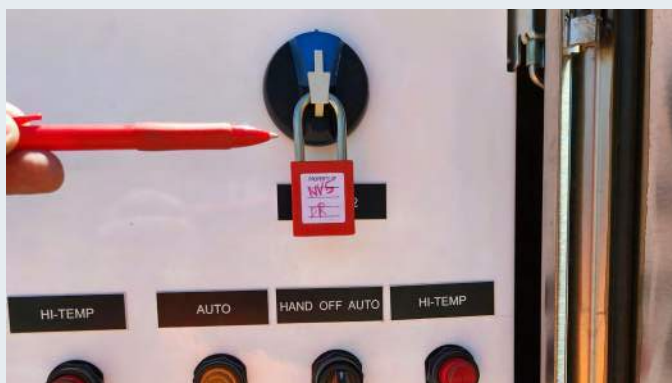
Example of Lock out tagout procedure for the Pump Well service.
