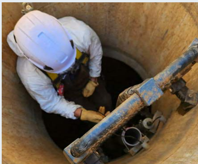
Underground service cleaning and inspection of Level loggers at Gates Canyon Project
