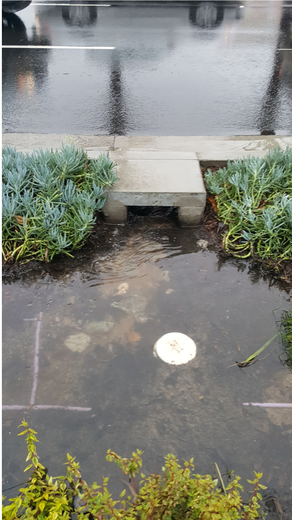
Figure B-2. Inflow to the Downey Bioswale during the January 12 Event.
