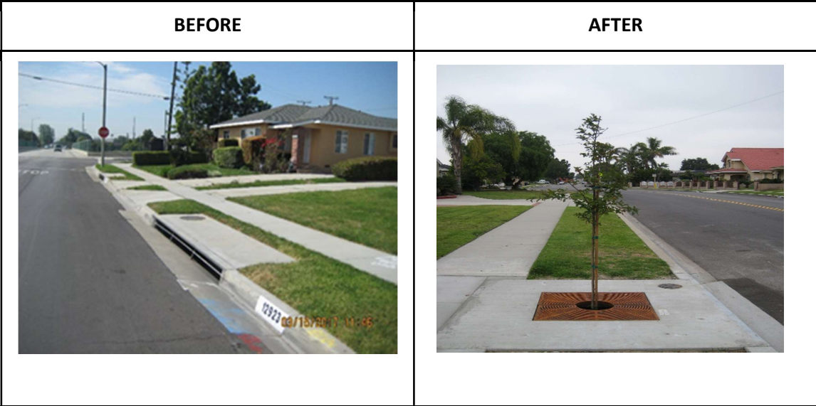
Tree Box Filter– 12923 Barlin Avenue (Downey)
