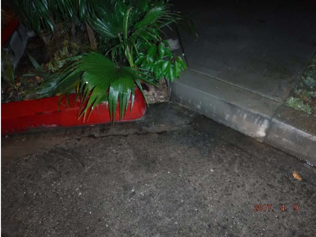
Figure B-21. Whittier Tree Well at 7751 Milton Ave during the April 8 Event.
