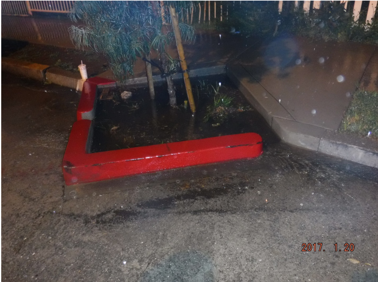
Figure B-17. Flow through the Whitter Tree Well at 7751 Milton Ave. during the January 19 Event.
