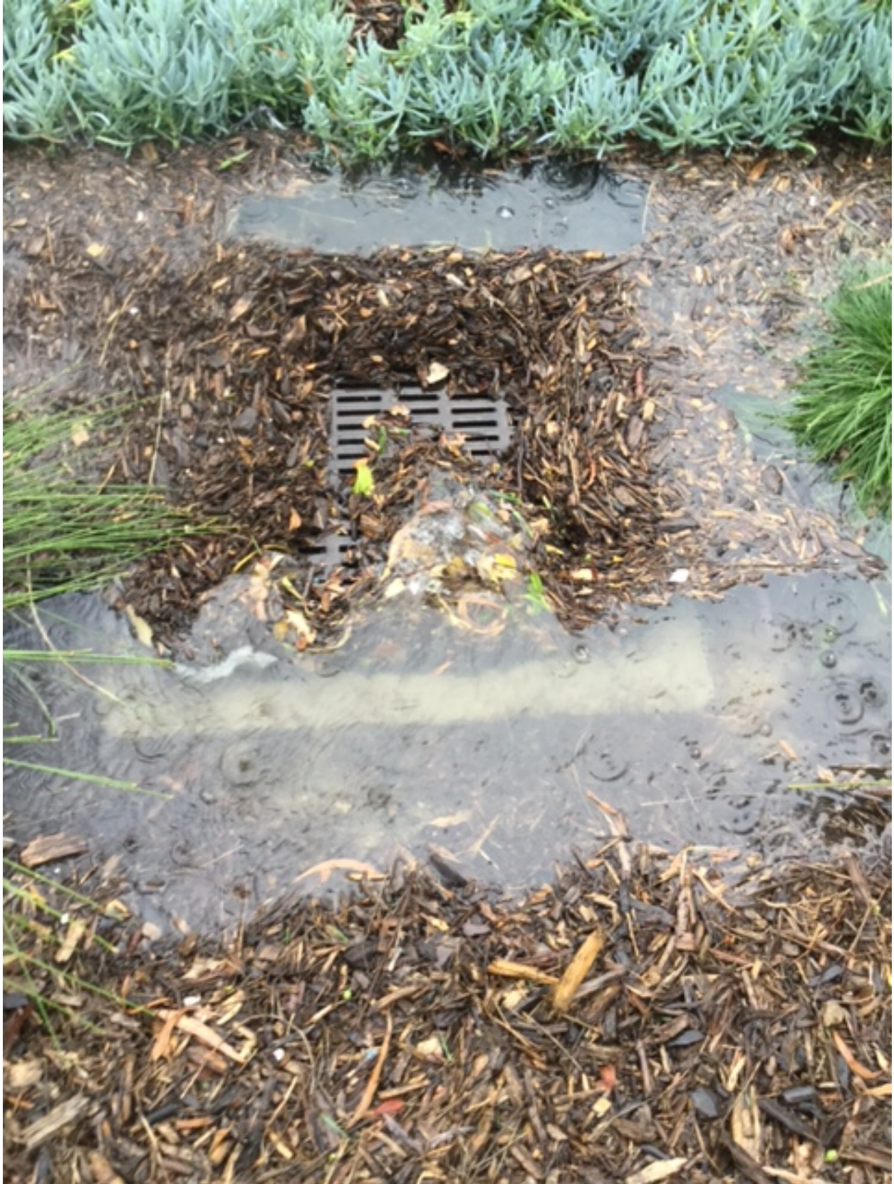
Figure B-7. Outflow from the Downey Bioswale during the February 17 Event.
