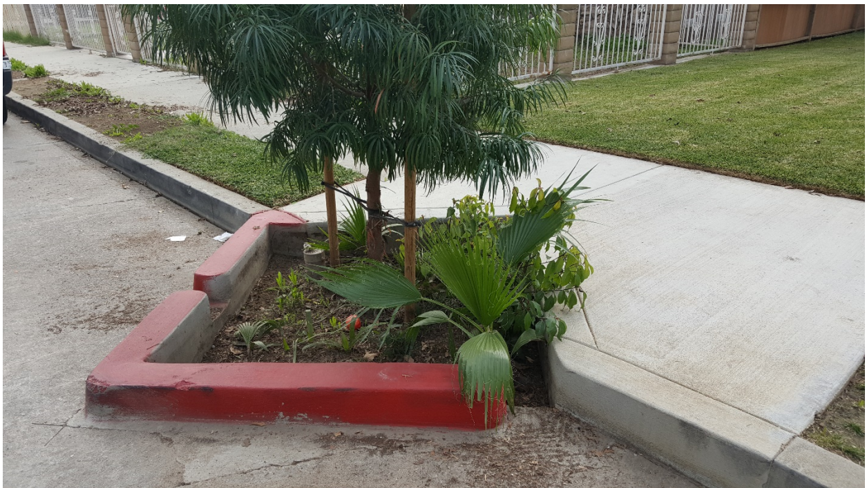
Figure B-13. Whittier Tree Well at 7913 Milton Street.
