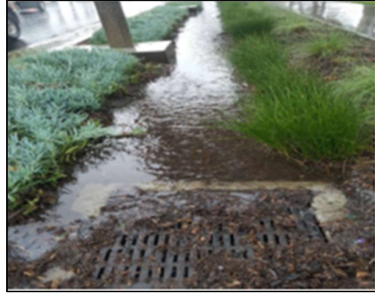
Bioswale stormwater outflow (February 17 th Storm Event)
