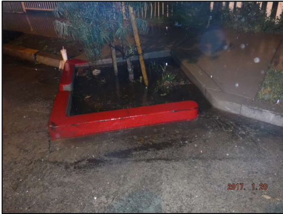
Bioretention Tree Well - 7751 Milton Avenue (January 19 th Storm Event)
