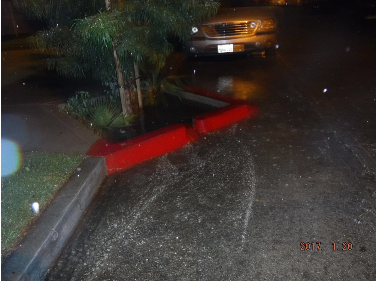
Figure B-20. Outflow from the Whitter Tree Well at 7913 Milton Ave. during the January 19 Event.
