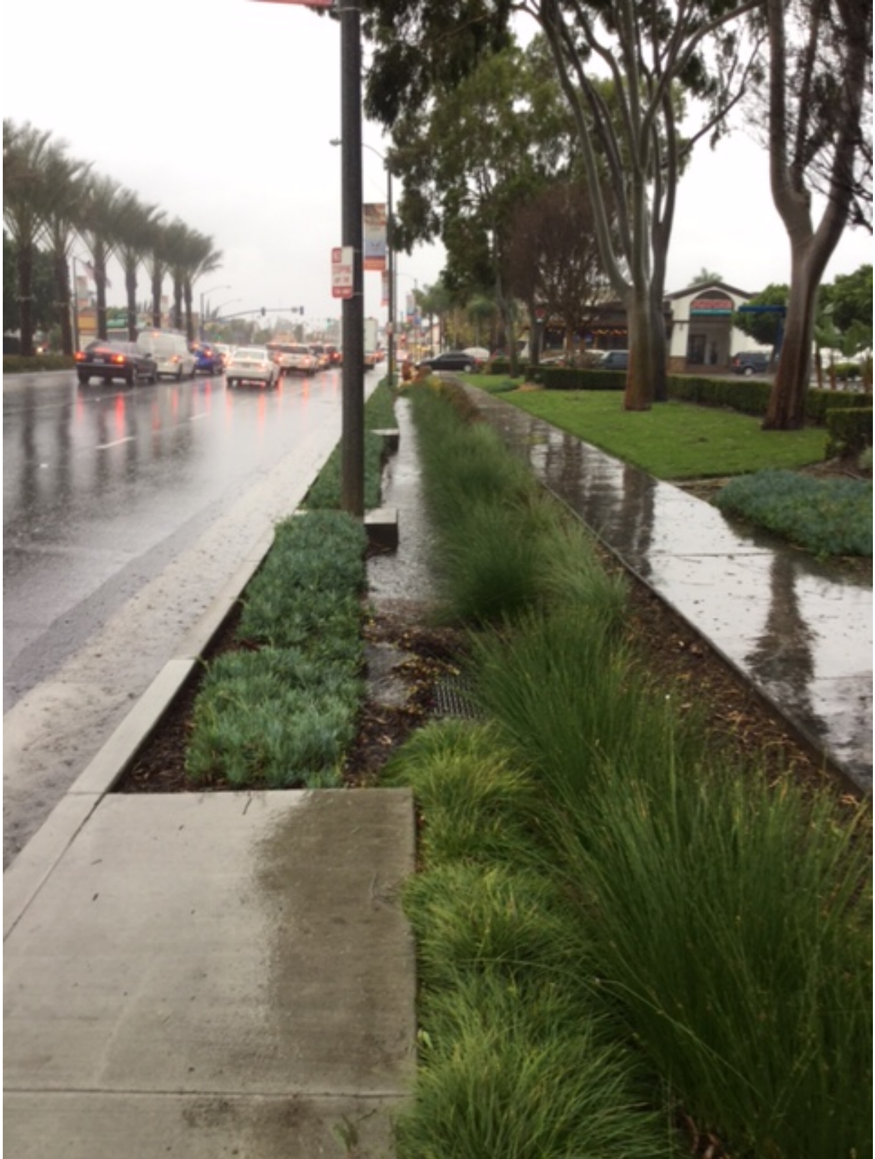
Figure B-6. Flow through the Downey Bioswale during the February 17 Event.
