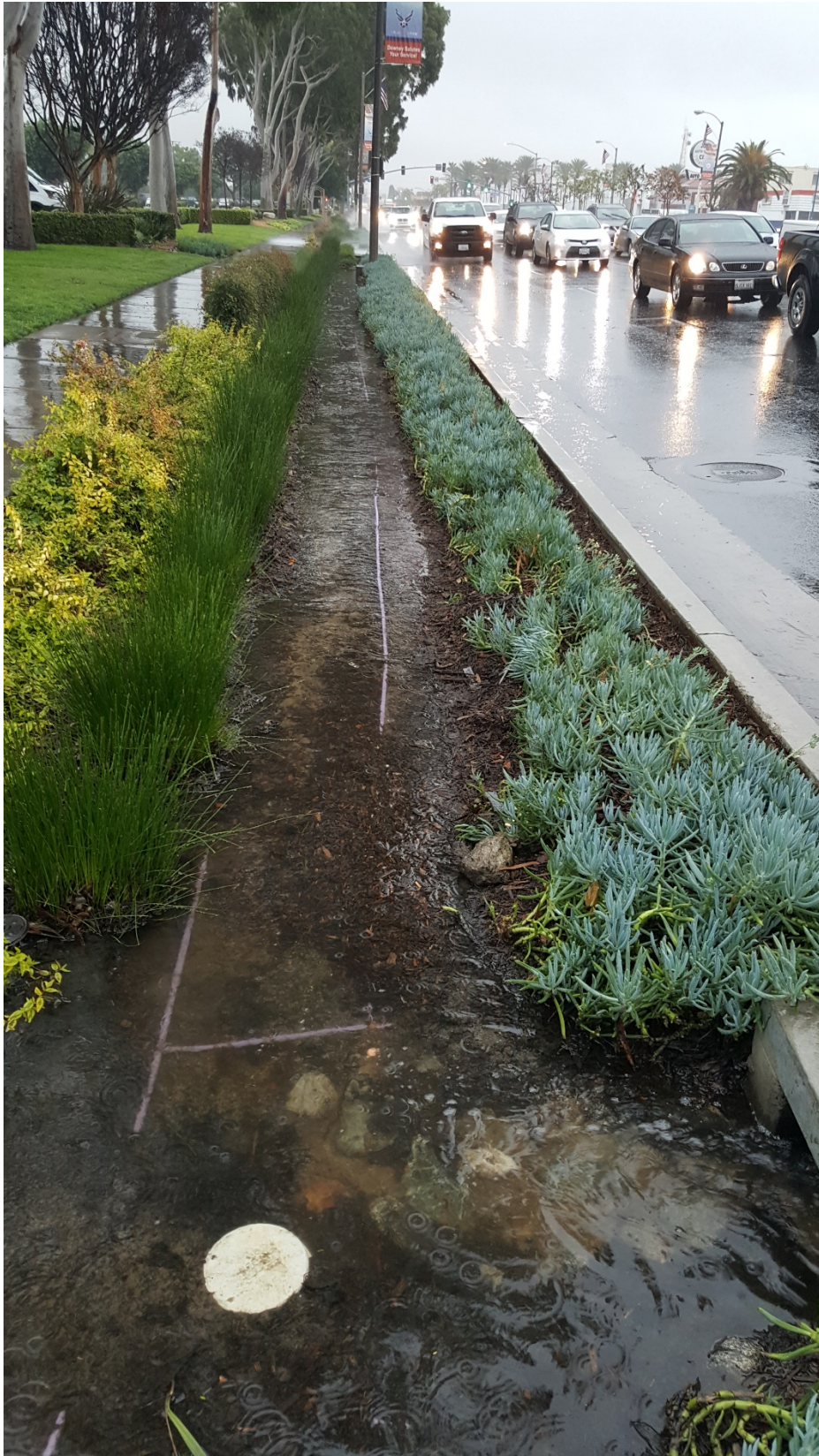
Figure B-3. Flow in the Downey Bioswale during the January 12 Event.
