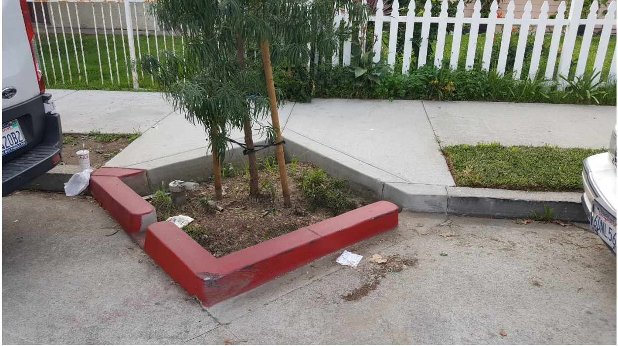
Figure B-12. Whittier Tree Well at 7751 Milton Street.
